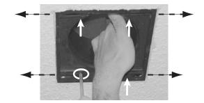
Insert Grill Assembly into the hole from the front. Fully extend and tighten the retro brackets behind the mounting surface.
