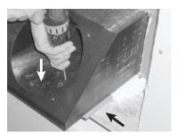
At the back, shim the vent outlet bottom to the correct height and screw the outlet body tightly & securely through the shim into the surface below.
