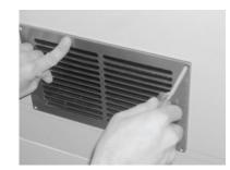
Insert the Vent Outlet & grill into the face of the hole; screw them firmly to the mounting surface using the 4 supplied screws.
