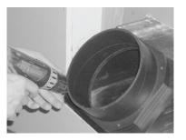
Attach the mounting flange to the back of the Outlet body using the supplied screws (4 for Silver / 5 for Mini).
