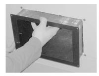
Press-fit the Vent Outlet through the front of the opening; mark the four screw hole locations.
