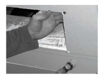
For drywall installs, remove the Vent Outlet and drill 4 holes sized for your fastener/anchors.
