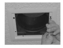
Using the four screws previously removed, screw the frame into the Outlet face, snugly sandwiching the mounting surface between the Grill frame and Outlet.
