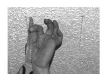
Using the supplied template, trace and cut a hole into face of the mounting surface.
